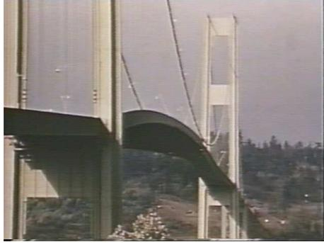
Figure 1: Tacoma Narrows bridge during self-excited structural vibration in 1940
