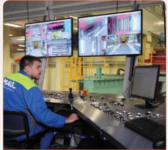
Inside the pulpit of the new rolling mill
